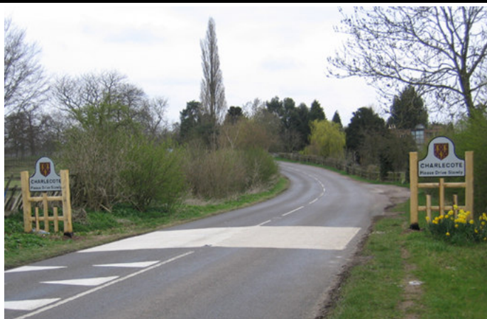
The new village signs and road markings at the entrance to Charlecote village
